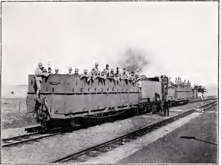
ARMOURED TRAIN NEAR ESTCOURT
